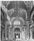
Massive groin vaults, as well as barrel vaults, were used in the basilica that was erected in the early 4 th c. by Maxentius and later acquired and completed by
